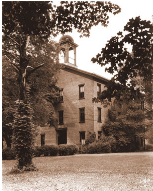
The new Main Classroom Building will stand on the spot where North Hall (above) first greeted Illinois Wesleyan students.
