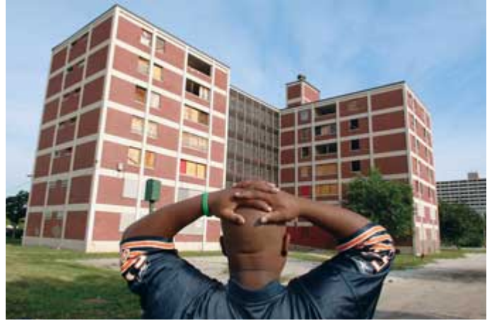
Sherrod takes in the desolate view at his childhood home, a public housing structure that now stands empty and will be demolished. With support from his mother and teachers, he was able to avoid the lure of gangs and drugs that consumed the lives of many in his neighborhood.
