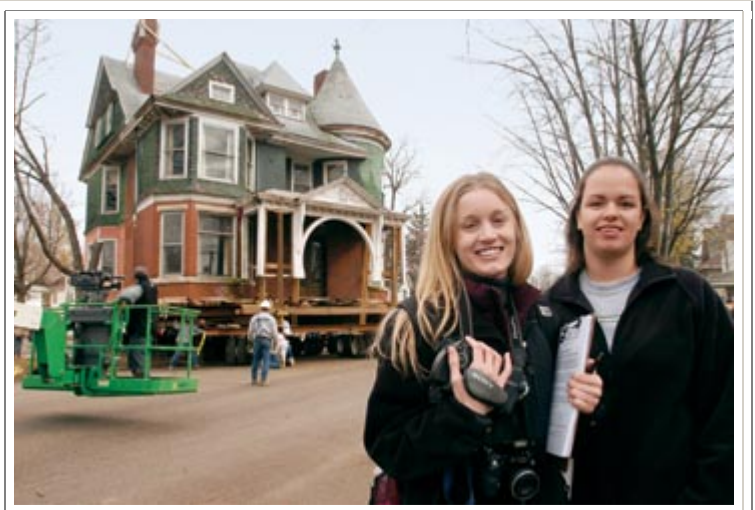
In their work with ARC, Maren Wesley '06 and Liz Jaroscak '06 (above) documented the seven-hour, two block journey of an 1894 Queen Anne-style house. Weighing an estimated 180 tons, the structure was moved in November by the Old House Society (OHS) , which helps restore and preserve historic homes in Bloomington. Wesley and Jaroscak helped OHS with pre-publicity and photographed and videotaped the move, collaborating with cable TV’s History Channel. (Photo by Marc Featherly)
