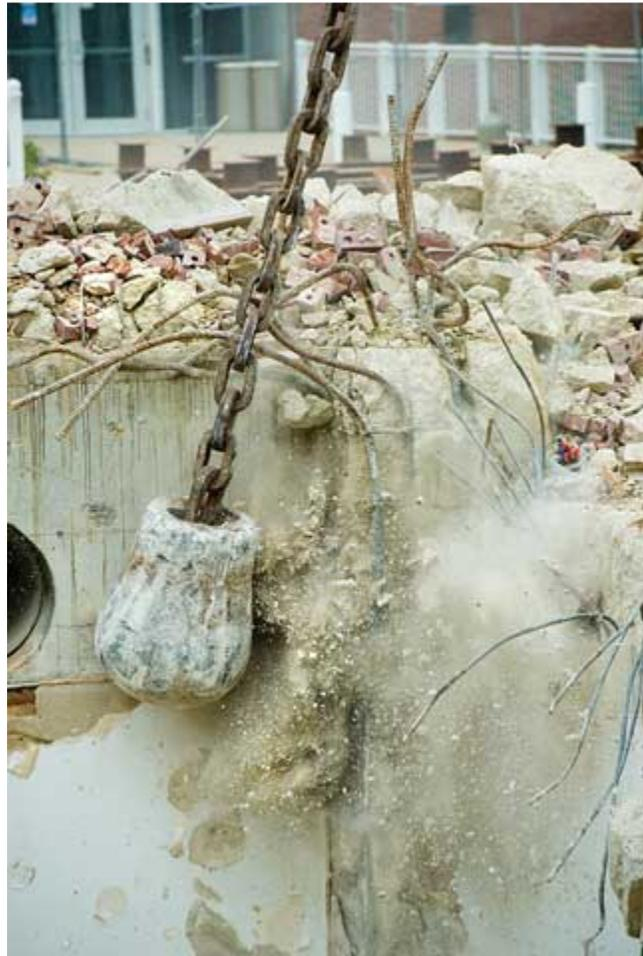
Sheean’s thick walls are smashed by a wrecking ball. Crushed concrete and brick will provide the new classroom building’s foundation. (Photo by Marc Featherly)
