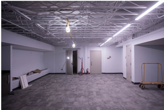
Construction is underway in the Underground of the Memorial Center.
