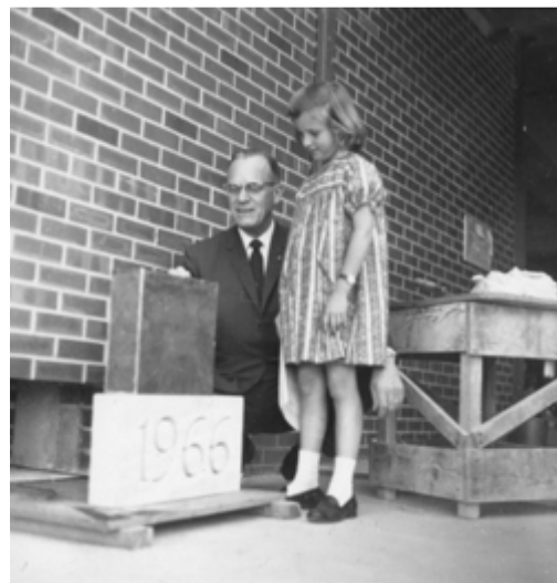
President Lloyd Bertholf kneels next to cornerstone of Sheean Library during a ceremony to place the time capsule in the building during construction. The young girl standing is the daughter of the building designer.
